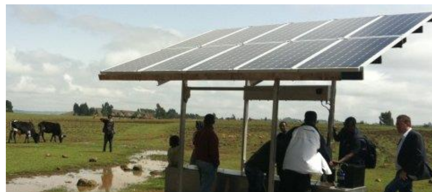
Solar-powered milk cooler in Ethiopia
