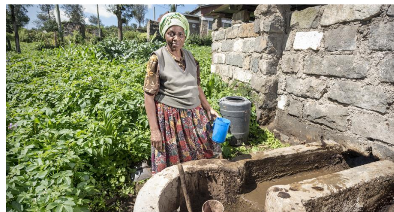
Kenyan dairy farmer next to her biogas digester, converting cow manure into fuel and fertiliser
